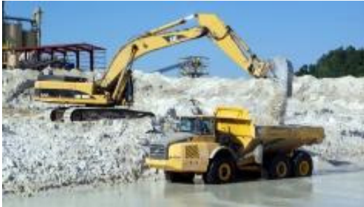
Onsite Mining / Excavation
