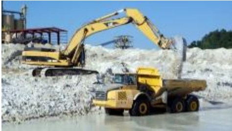
Onsite Mining / Excavation
