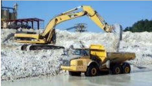
Onsite Mining / Excavation
