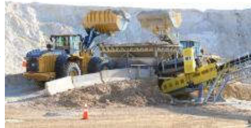
Conveyer Belt to Onsite Wet Plant
