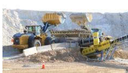
Conveyer Belt to Onsite Wet Plant
