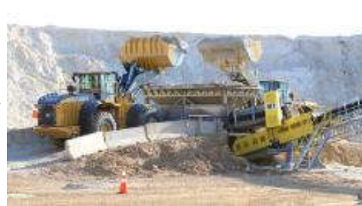
Conveyer Belt to Onsite Wet Plant
