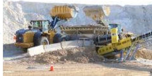
Conveyer Belt to Onsite Wet Plant
