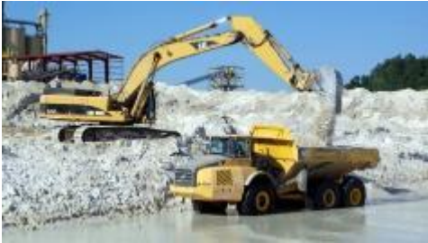
On-site Mining / Excavation
